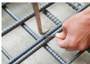
Manual operation using pliers
