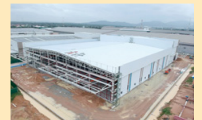
TIE WIRE production factory under construction
