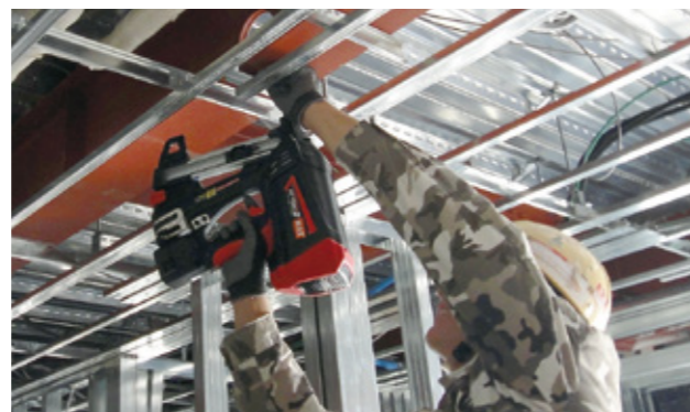
Cordless gas-powered pin-driving tool "Gas Nailer"
